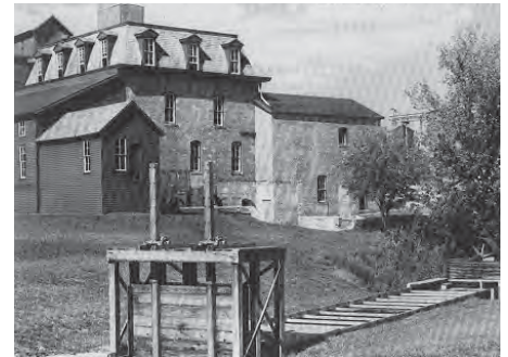
Neligh Mills, one of the first structures in Neligh, as it appears today.
