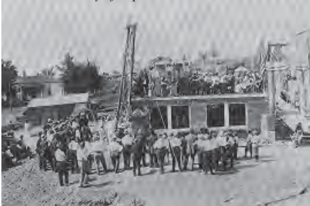
Laying cornerstone for Neligh High School, 1913. Photo courtesy of http://www.casde.unl.edu/ .
